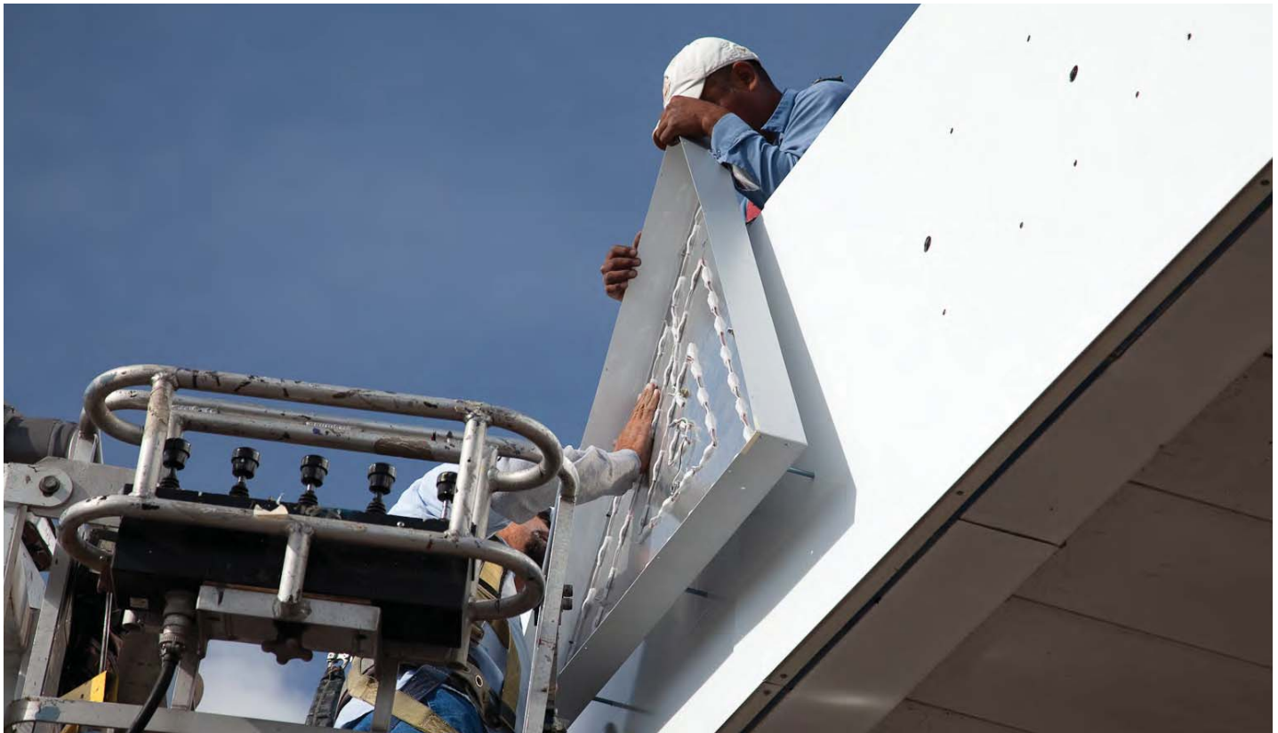
Installing the Trimark.
