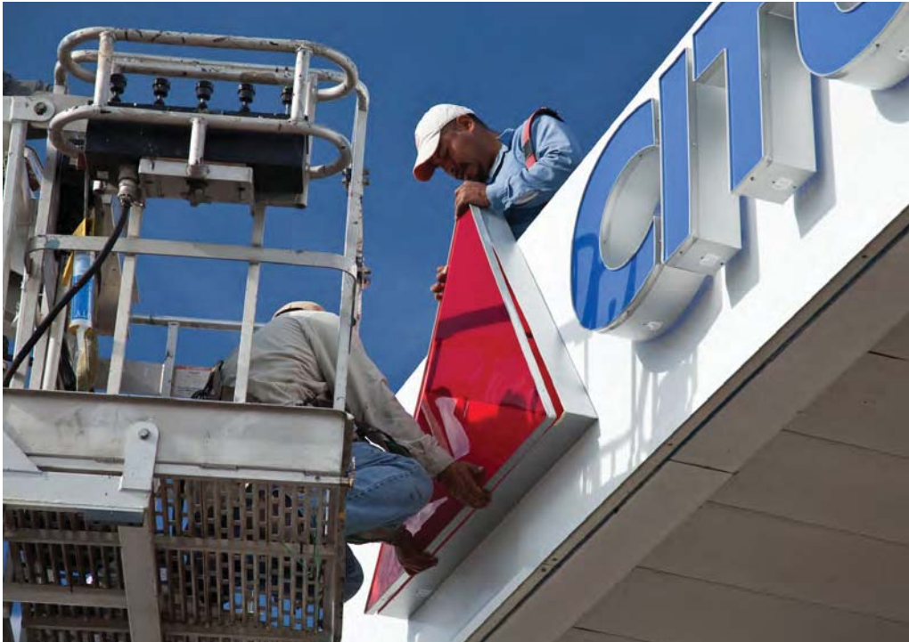
Installing the Trimark and channel letter faces.
