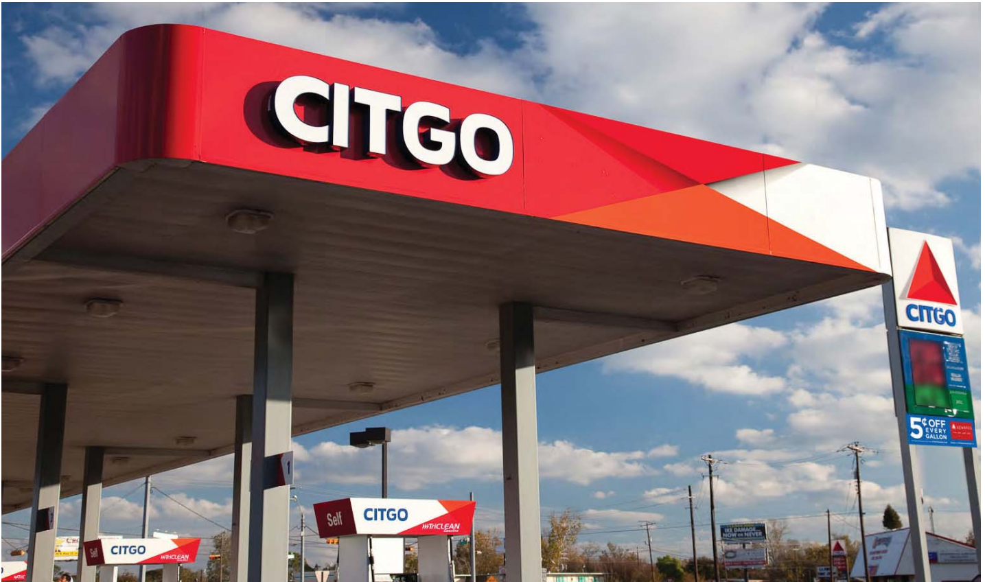
Completed secondary side of canopy with white CITGO channel letters. Note that the secondary side is 65% red and 35% white.
