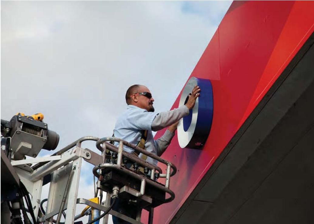
Installing the secondary white channel letters on the canopy.
