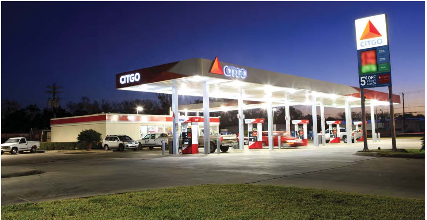
Completed image (nighttime). Note the halo on the primary blue CITGO channel letters.
